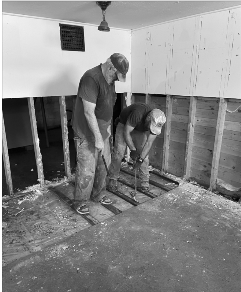
Ben Williams and Chris Koteas remove flood-damaged walls and flooring from the Town Office basement. (photo by Robin Durkee)
