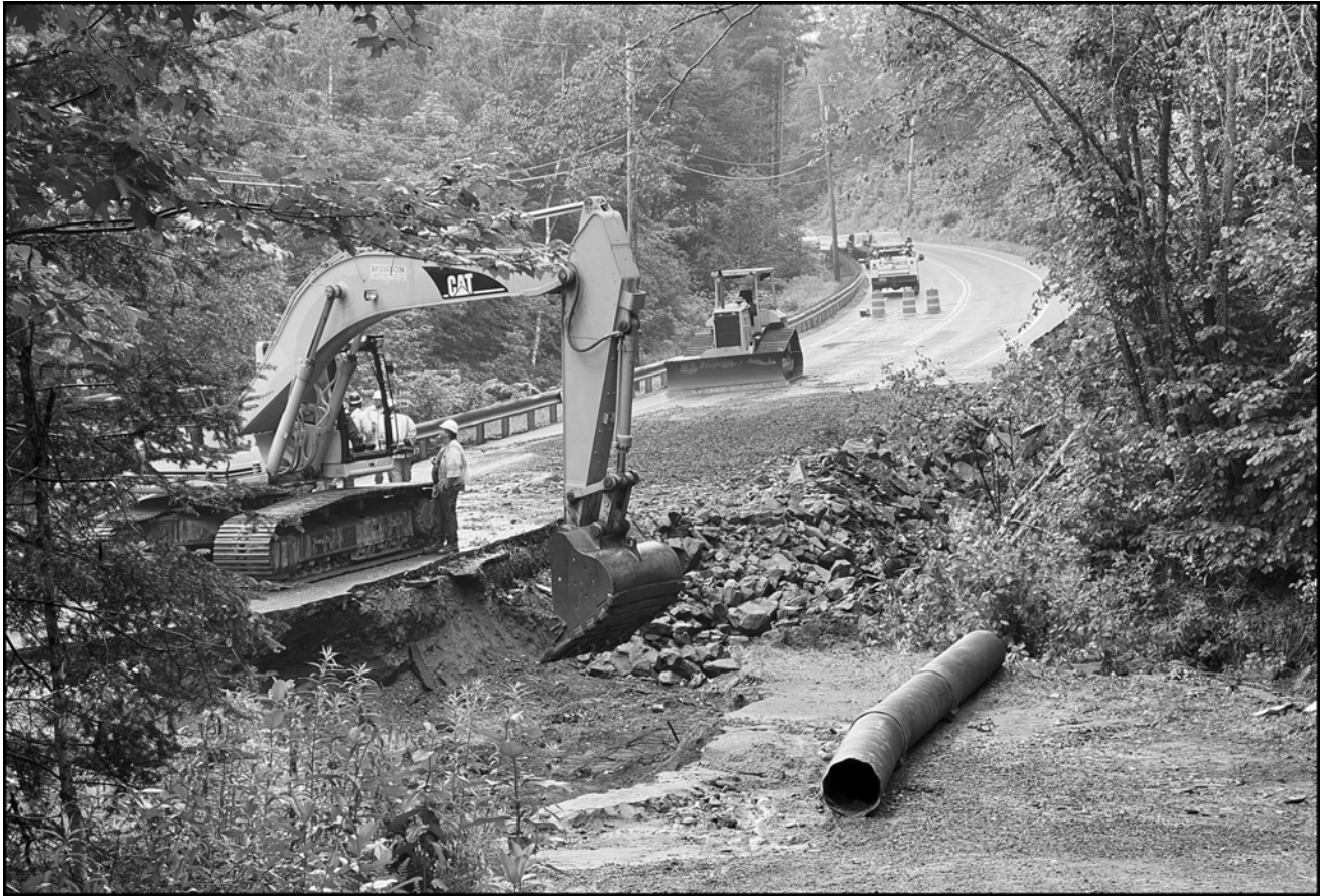
Rebuilding a stretch of Vermont Route 14. Portions of the highway were washed out – pavement and road bed, gone – north and south of Woodbury village, in the July flood. (photo by Jayme Lowell)
